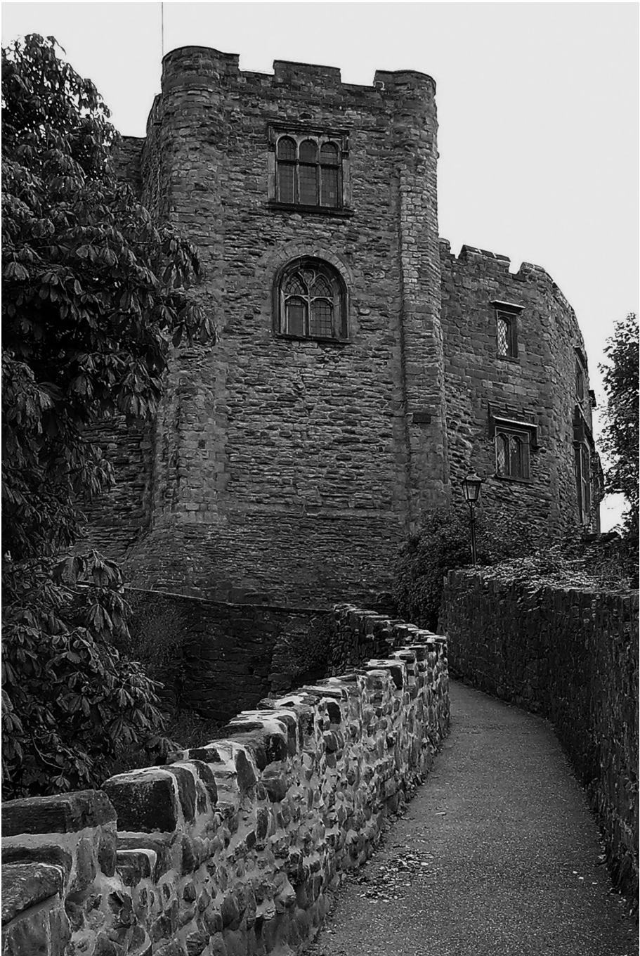
Tamworth: Approach to the shell keep (C12 and C13).
